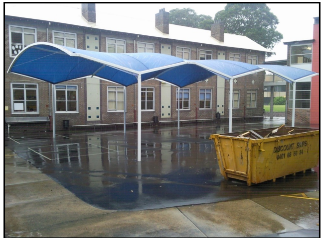
The new shade structure providing Year 7 students with a sun-safe play area at recess and lunchtime.
